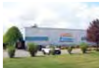
UST Chicopee Plant
